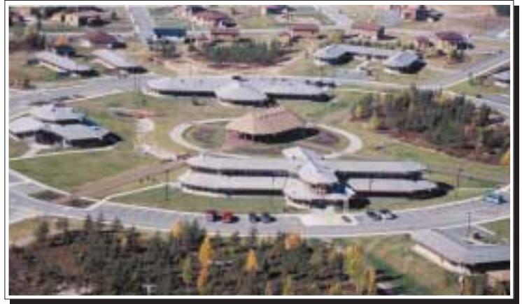
Community buildings in Ouje-Bougoumou. From now on, the Crees will have responsibility for developing new infrastructures.
