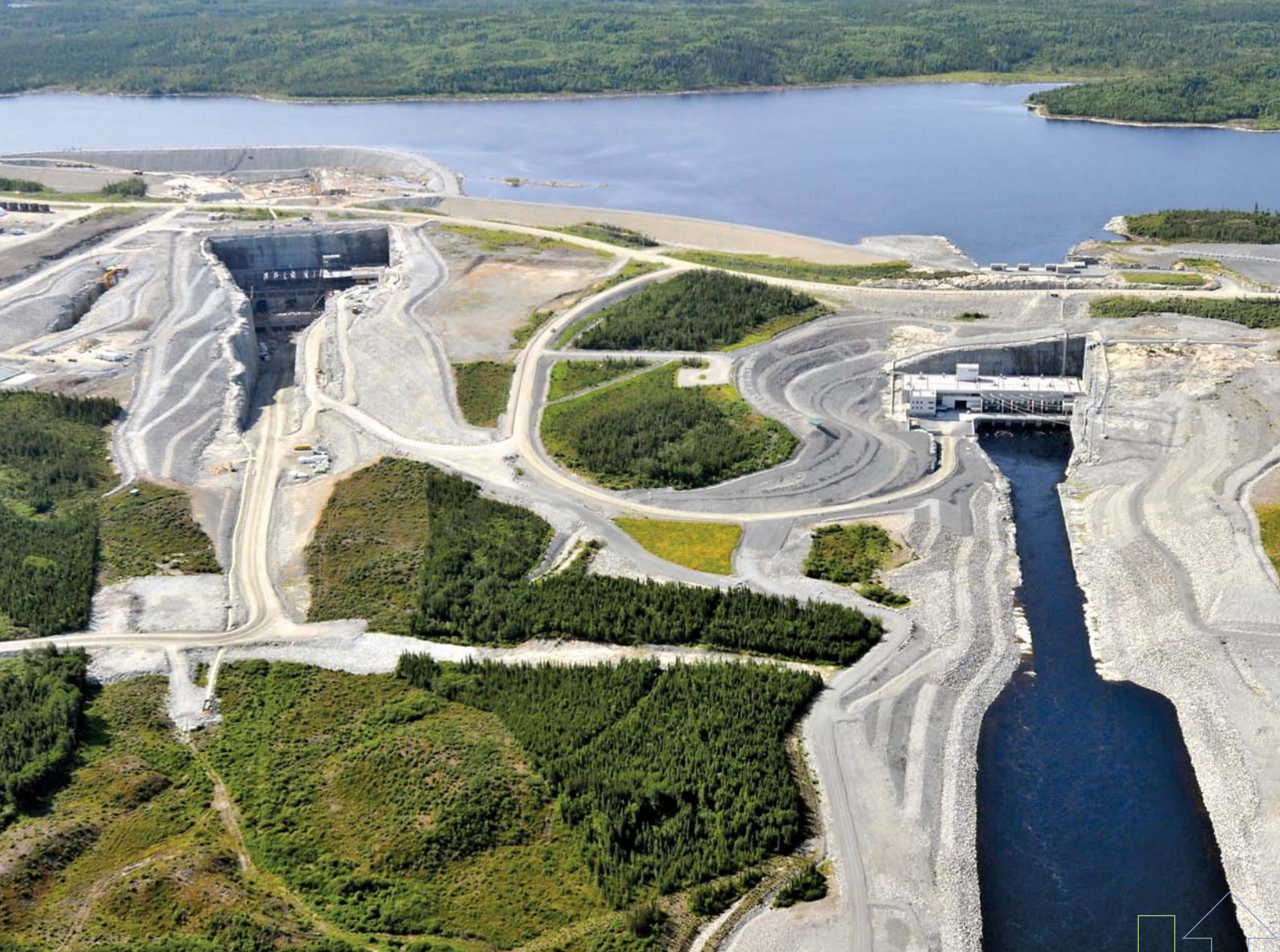
Eastmain-1 powerhouse and Eastmain-1-A construction site
