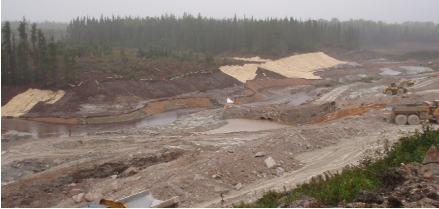
The Barvue site, creek diversion work.
