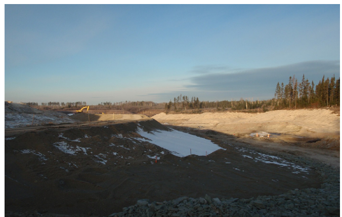
The Barvue site, berm construction.
