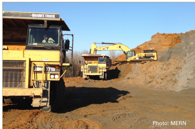
Excavation of mine tailings at pond B.
