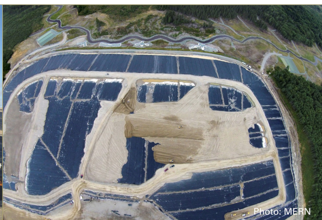
Rehabilitation work at the Barvue site.
