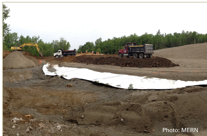
Beginning deposition of waste rock in the containment cell.
