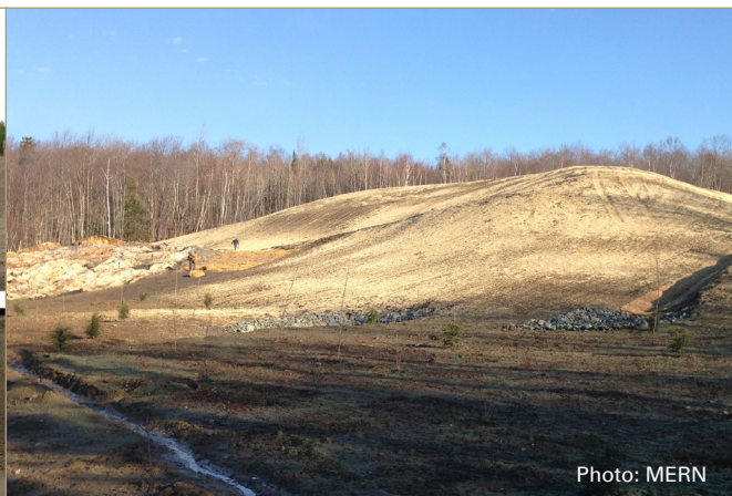
Waste rock cell after completion.
