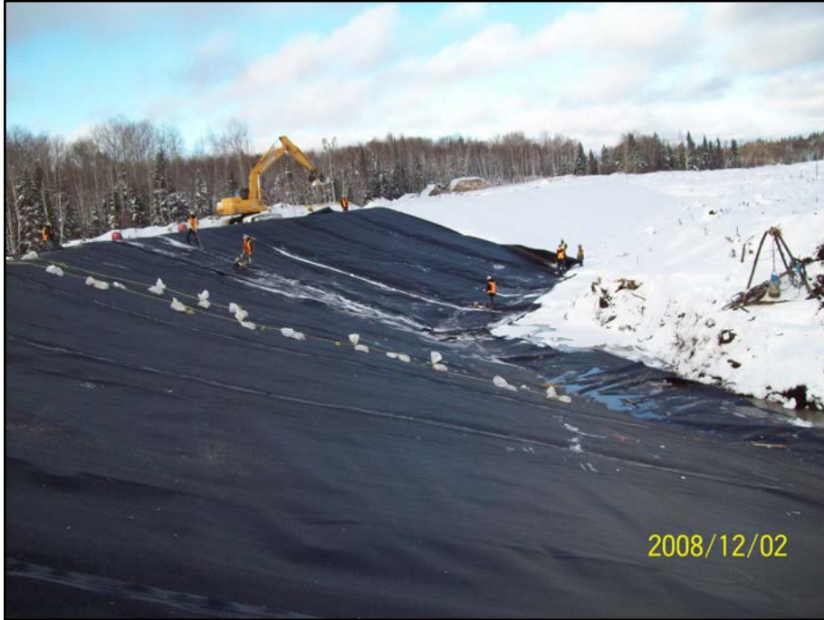
Photo 5.15 : Digue F – Installation géomembrane
