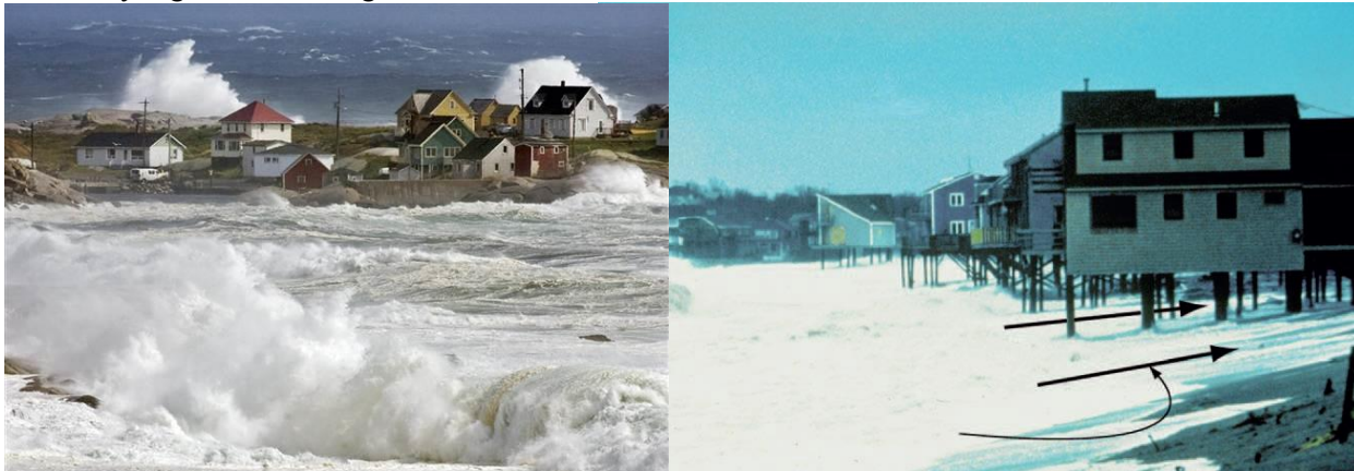
Figure A.7. (Left) Storm waves breaking at Peggy's Cove, Nova Scotia during Hurricane Earl on September 4, 2010 (Andrew Vaughan-The Canadian Press). (Right) Wave runup beneath elevated buildings at Scituate, MA, during the December 1992 nor'easter storm (USFEMA, 2011)
